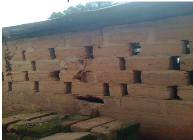
Fig. 3: Poultry house constructed with block masonry
