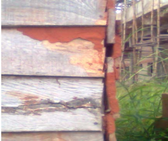
Plate 4: Termite Infested Wooden Structures
