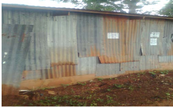
Fig. 2: Poultry house constructed with corrugated roofing sheet
